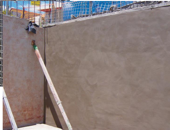
Above: Finished shotcrete walls.
