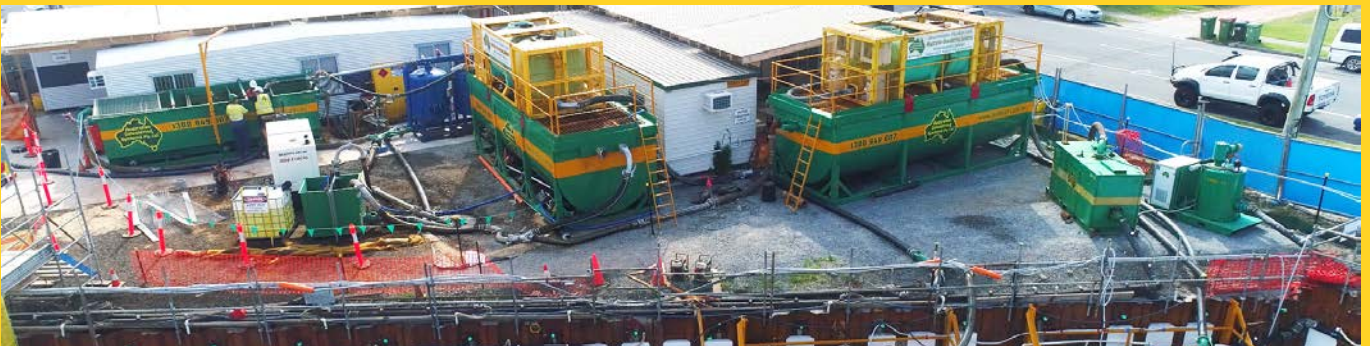
(Water being discharged from site after being processed through Heavy Metal Treatment System)
