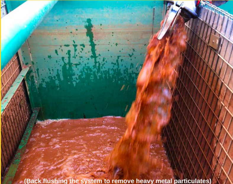
(Back flushing the system to remove heavy metal particulates)
