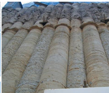
Bottom right: SMW used as a boundary retention system.
