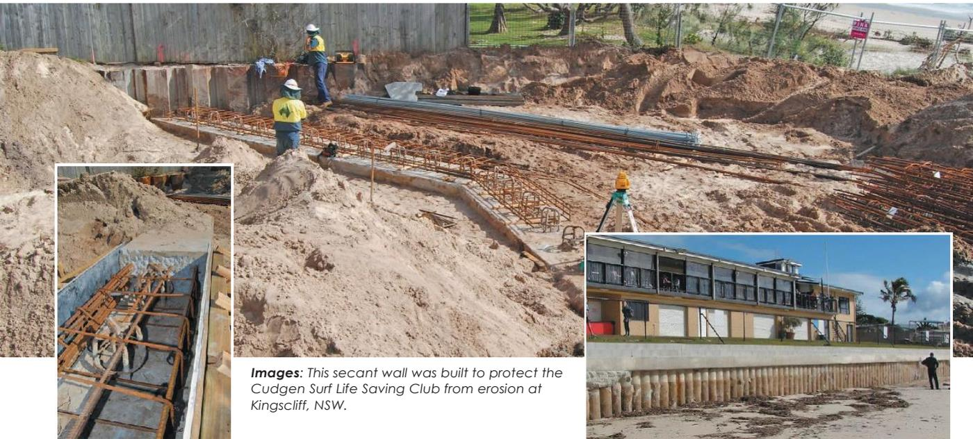
**Images:** This secant wall was built to protect the Cudgen Surf Life Saving Club from erosion at Kingscliff, NSW.
