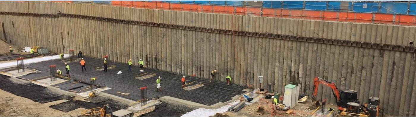
Secant piling is an ideal solution to create a retaining wall which inhibits the passage of water and is particularly effective where groundwater control is complicated by stratified ground. Popular applications include beachfront scour protection walls and basement 'groundwater cut-off' walls.
