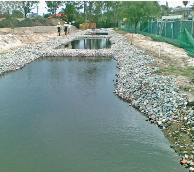
Above: Groundwater filtration tank.
