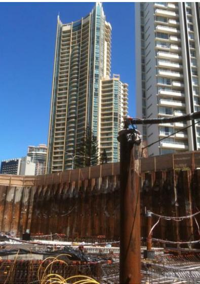
Deep well dewatering is recognised as a cost effective and efficient way for medium to long term dewatering of larger projects where the excavation is greater than 4m or when a wellpoint system is deemed inefficient.
