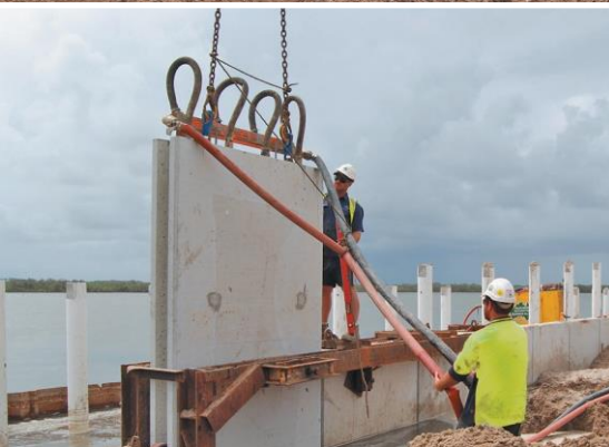
Above right: The water jetting head attached to the top of the panel prior to lifting.
