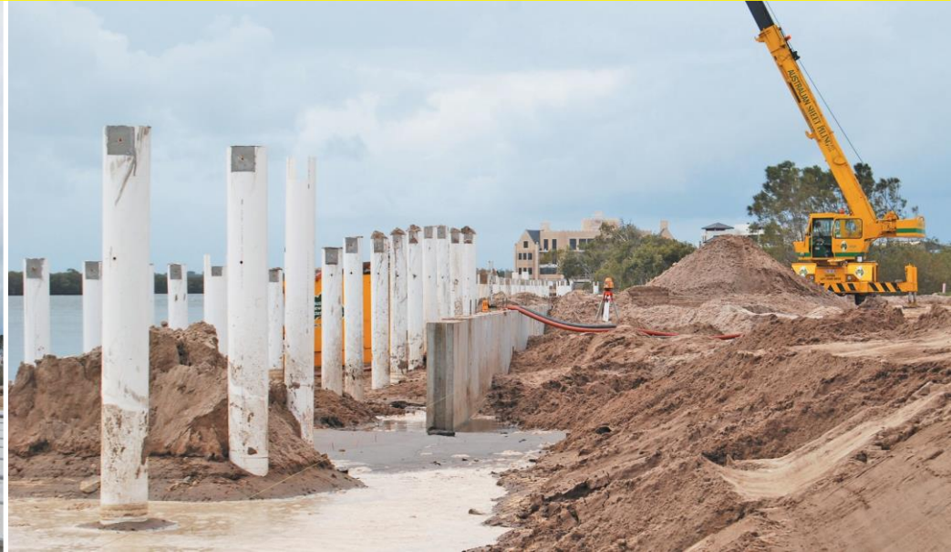
Above: Partially completed revetment wall with dewatering taking place between the wall and the temporary line of sheet piling. The top edge of the wall is finished with capping beams. Left: Lifting a panel to the revetment line. The capping beams that top the wall can be seen in the foreground.
