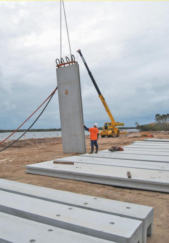
Above: Partially completed revetment wall with dewatering taking place between the wall and the temporary line of sheet piling. The top edge of the wall is finished with capping beams. Left: Lifting a panel to the revetment line. The capping beams that top the wall can be seen in the foreground.
