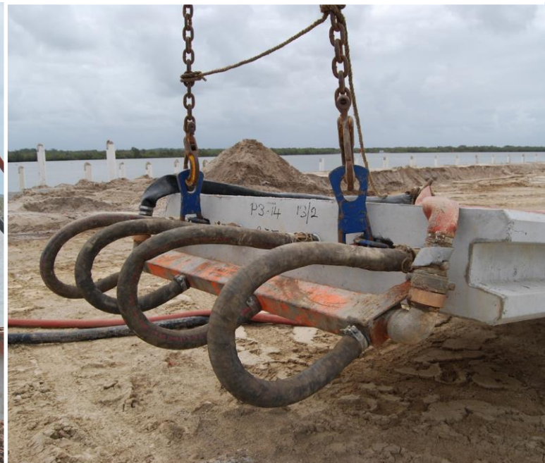
Above: Partially completed revetment wall with dewatering taking place between the wall and the temporary line of sheet piling. The top edge of the wall is finished with capping beams. Left: Lifting a panel to the revetment line. The capping beams that top the wall can be seen in the foreground.
