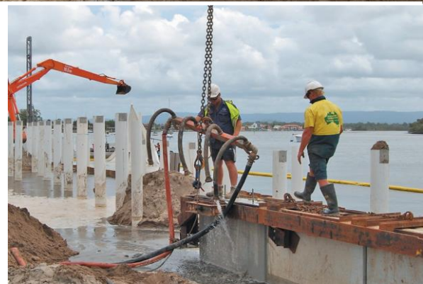
Above right: The water jetting head attached to the top of the panel prior to lifting.
