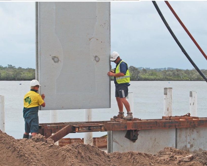
Above: Partially completed revetment wall with dewatering taking place between the wall and the temporary line of sheet piling. The top edge of the wall is finished with capping beams. Left: Lifting a panel to the revetment line. The capping beams that top the wall can be seen in the foreground.
