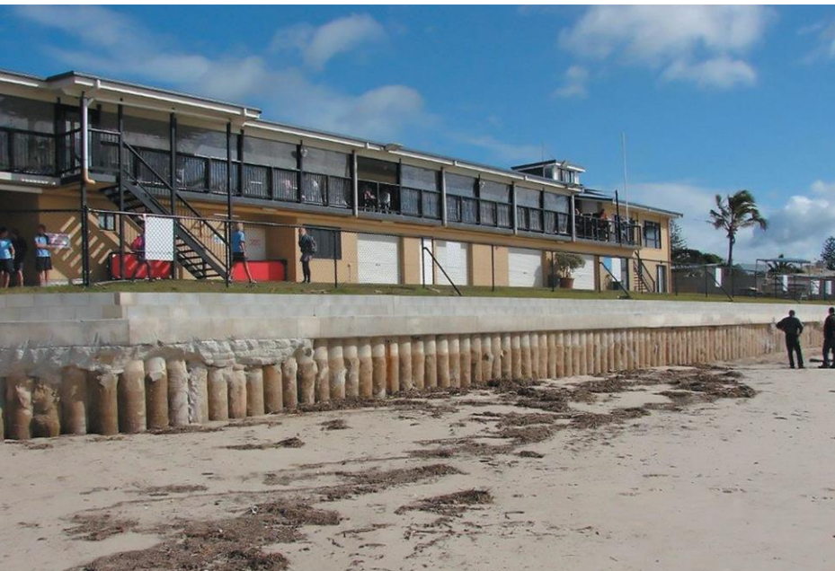
Above: CFA piles form part of this secant wall at Cudgen Surf Life Saving Club that has saved the building from erosion by the ocean.
