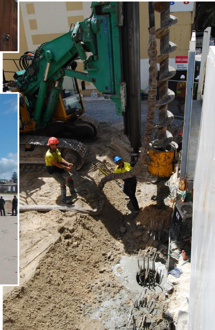
Below: CFA installation on a site bounded by neighbouring buildings and a highly trafficked roadway.
