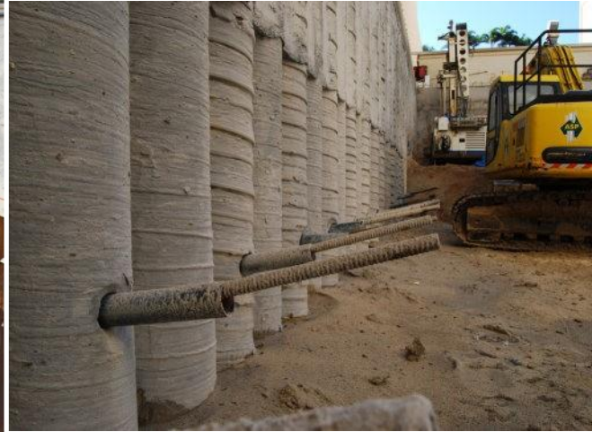
Below: CFA installation on a site bounded by neighbouring buildings and a highly trafficked roadway.
